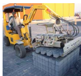
VM-203: Shifting rectangular pavers into running bond
