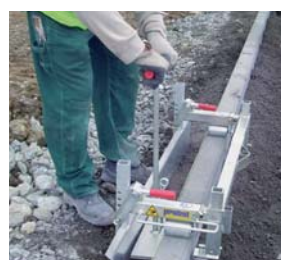
Slipform for Concrete Kerb Backfill GR-150
