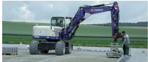
HVZ-GENIUS Hydraulic Installation Clamp in combination with excavator
