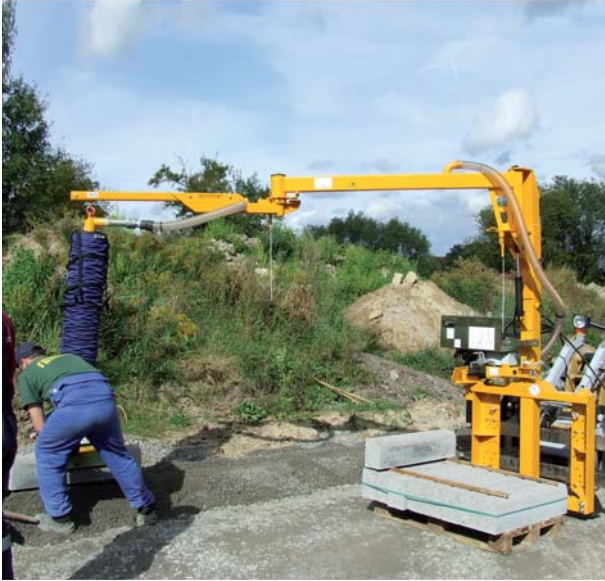
JUMBO-BV-VARIO Vacuum Kerb Stone Installation
