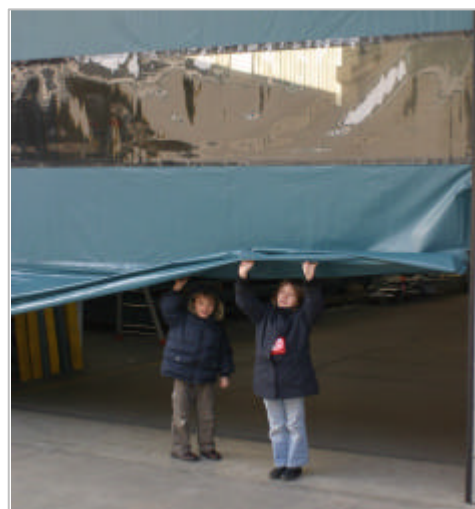
The mass descending on possible obstacles is so insignificant that there is no need of safety rib.
